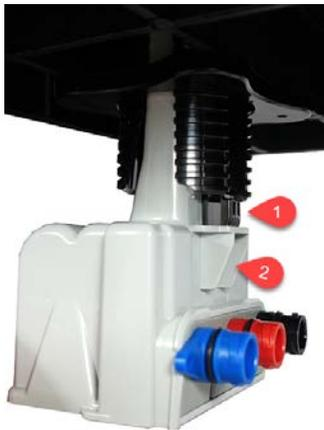
4. Verify that the clip locks into place and the retainer clip collar is hand-tightened against the pit lid.
